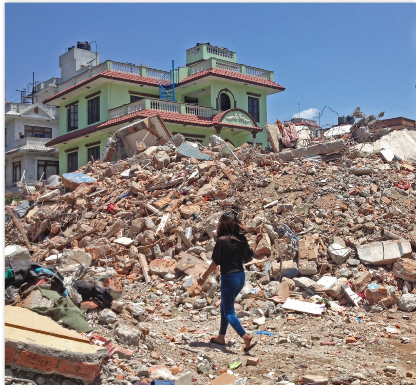
Figure 1.1 Earthquake destruction in Kathmandu, Nepal. The April 25, 2015 earthquake toppled many culturally significant buildings and caused 9,000 fatalities and US$4 billion in damage. Natural disasters are tragic reminders of the close relationships between human societies and the natural environment. © Michelle Fyneweaver.
